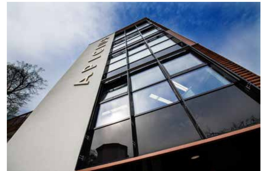
A total of seven kitchens, spread over six floors
